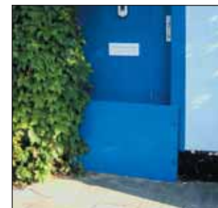
Flood-board on front doorway
